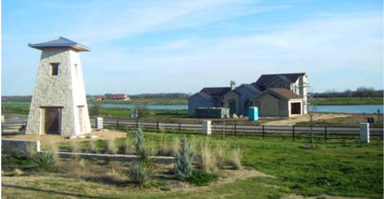
Above: Home Construction Continues at SMRR
